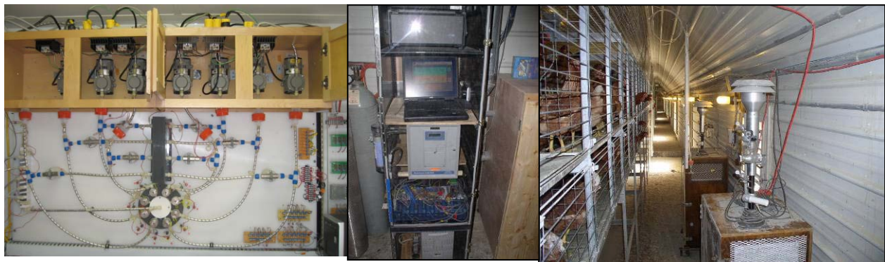
Figure 3. Gaseous and particulate matter (PM) concentration monitoring system (L- R: positive-pressure gas sampling system or P-P GSS, gas analyzers, and Tapered Element Oscillation Microbalance or TEOM PM monitors).
